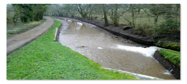
A finished stretch of installed Nicospan and back-filled with dredged silts.
