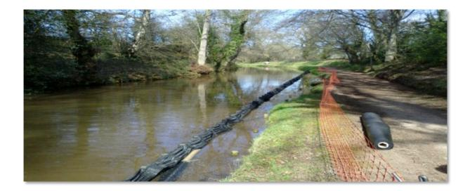
Tencate's Geolon PP15, a medium-strength woven geotextile is then installed at the rear of the Nicospan, the geotextile is folded over and placed along the edge of the front posts and stapled down with 40mm x 4mm galv steel staples, giving a neat front edge finish. The geotextile acts as a separator and holds the silts in place; it is installed across the back of the repair and slightly up the back of the bank.
