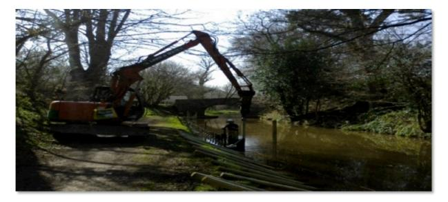
On this section of canal the wider towpath enabled Land & Water Services to use a digger with a hammer attachment and cup to knock the posts down.
