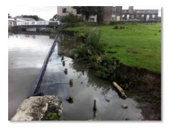
Nicospan is a prefabricated; double weave revetment fabric manufactured from strong UV stabilised monofilament yarns with pockets. Each pocket is 220 mm wide to allow 100 mm (max) diameter posts to be used as fixings.
