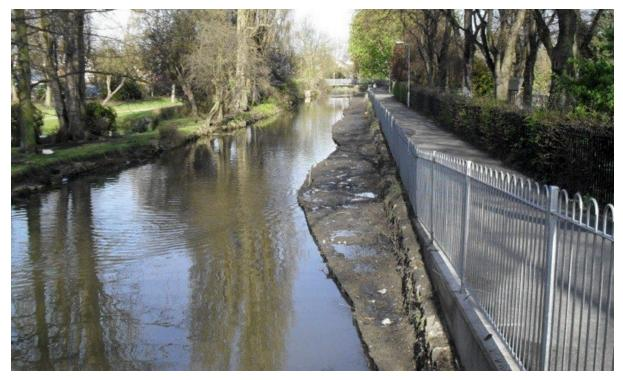
The river has now been fully dredged and all the silts have been retained on site and used within the Nicospan system which is now ready to receive the pre-planted coir pallets.
