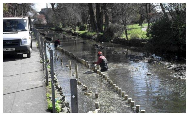
Nicospan is installed to form the required ledge shapes and to create the vertical faced revetment. The posts are cut down to the correct levels. A back line of 1.8m long x 100mmØ FSC posts are installed 1.5m behind the front posts, the two sets of posts are tied together, using a galvanised steel wire, to bring strength and stability to the system.
