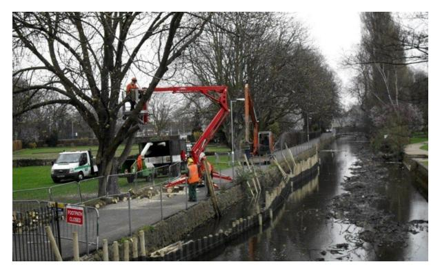
The scheme is lined out and the Nicospan installation begins, 2.4M long FSC posts are put into the pockets of the Nicospan and driven into the silt using a hammer attachment on the excavator. As part of the scheme overhanging tree branches were trimmed back to help reduce the organic matter, leaves, branches from dropping into the river system.
