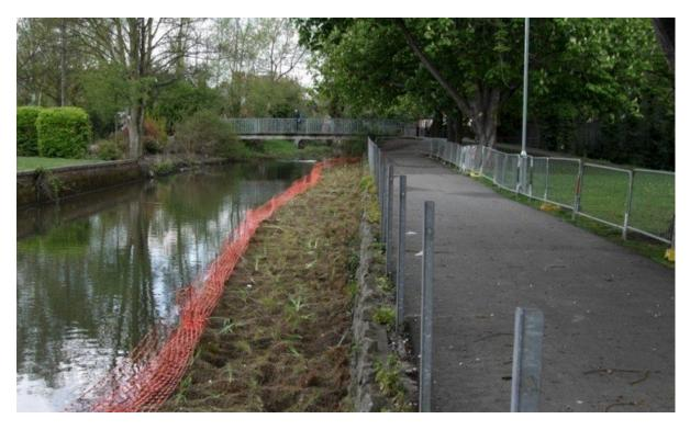
The coir pallets are fully installed into the Nicospan system, in time a fully vegetated edge will develop, the ledges will provide a natural habitat system for the local wildlife. The system gives a long lasting, aesthetic and environmental result.
