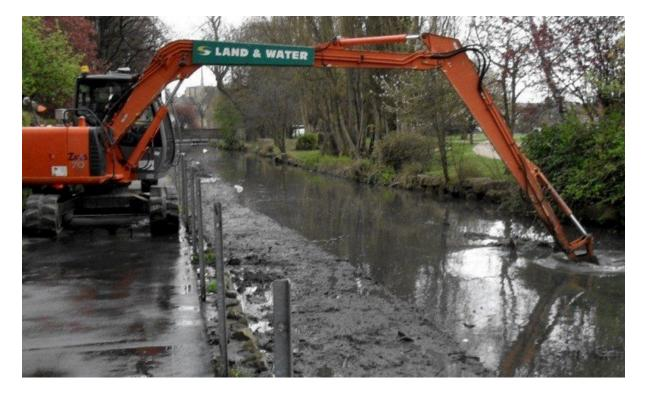
Dredged silts are used to fill in behind the Nicospan system and create the foundation for the ledges. The fertile silts will provide an excellent growing medium for the soon to be laid preplanted coir pallets. The established root systems of the plants, within the coir pallets, will soon grow down into the soils taking out excess moisture and quickly stabilise the soil ledges.
